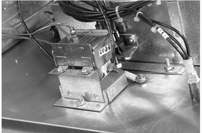
22. Connect wires labeled 'HT' to hi-limit thermostat terminals.
