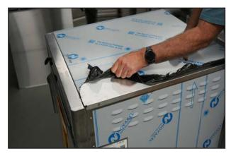
2. Locate the new top in the kit and place the top on the bottom unit. Peel the protective film off the top.
